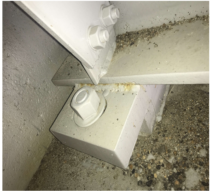
PHOTO 2 Description Span 1 bent 1 lack of fusion of weld from bottom of girder 8 to sole plate
