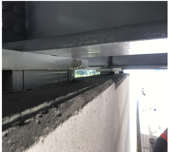
PHOTO 2 Description Bent 3 bearings paint flaking typical of bearings on this bent.
