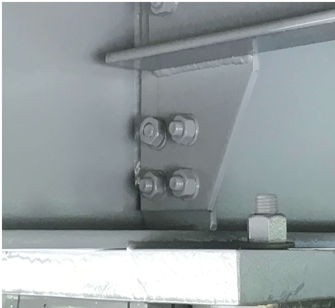
PHOTO 1 Description Bent 2 between girders 4 & 5 diaphragm 1 loose bolt
