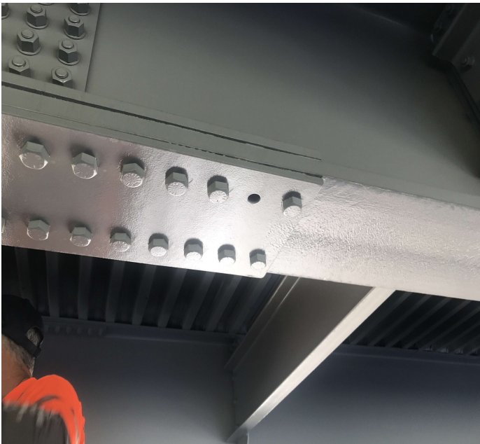
PHOTO 1 Description Span 3 splice 1 girder 3 missing bolt.
