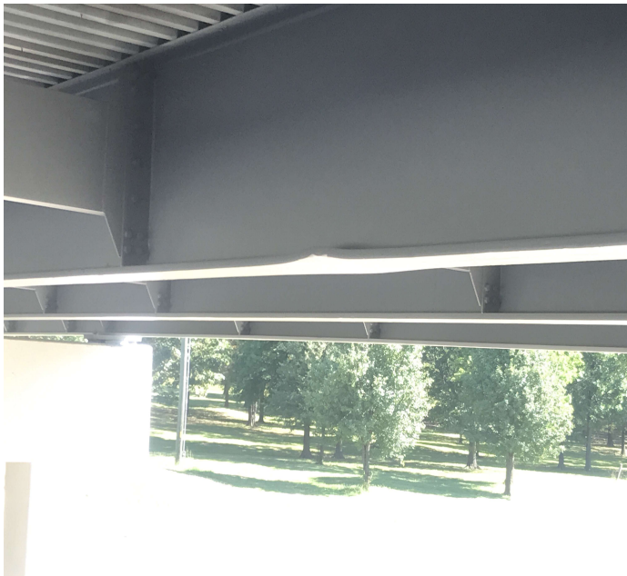
PHOTO 1 Description Span 2 girder 8 old impact damage over outside lane.
