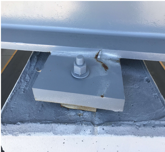
PHOTO 1 Description Bent 3 left side rust on bearing. Photo to monitor.
