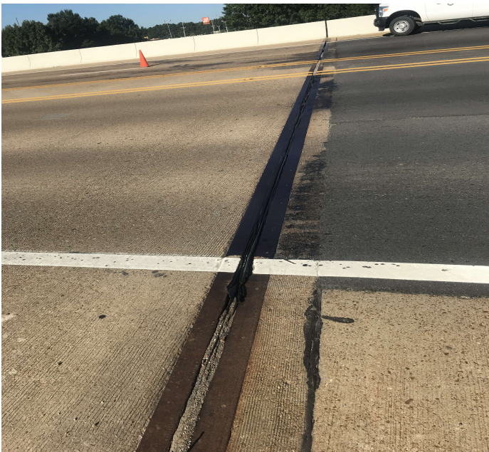
PHOTO 1 Description Both joints seals have almost complete failure.
