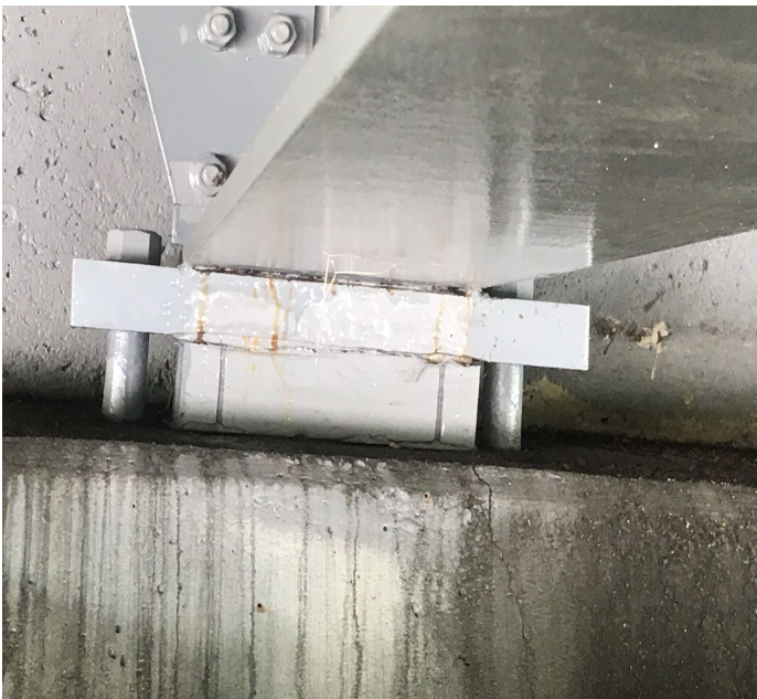
PHOTO 1 Description Span 1 bent 1 girder 5 pack rust forming between girder and bearing.
