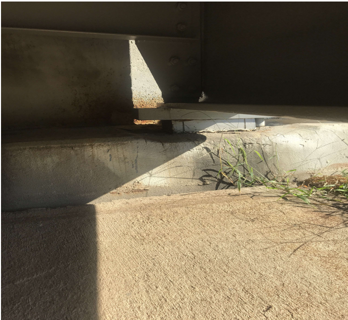
PHOTO 1 Description Span 4 bent 5 bearing under girder 10 on left side has missing anchor bolt.
